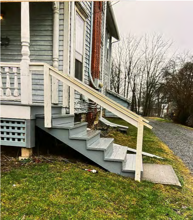
219 Clinton Street Side Porch
